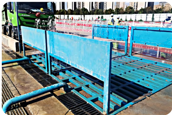
▲ Sedimentation Tanks and Vehicle Washing Facilities at the "Grand Canal Data Port ESG Innovation Center Project" Site
